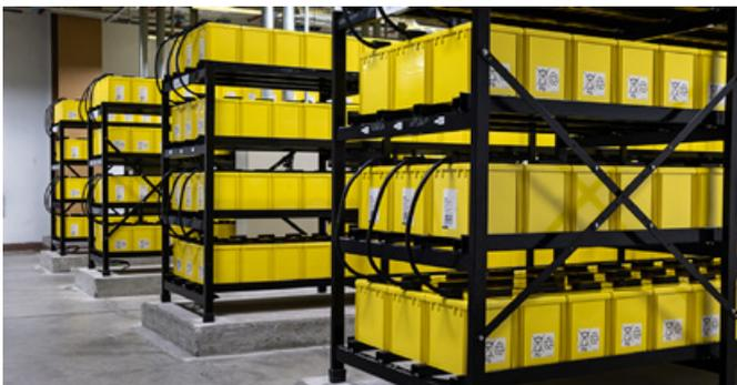
and easy to transport, handle and recycle. Crucially, advanced TPPL technology significantly improves energy efficiency, by providing up to 43% energy reduction compared with traditional VRLA batteries through reducing float current requirements. Further energy savings accrue as it can operate, within warranty, at elevated temperatures, reducing air-conditioning requirements.
