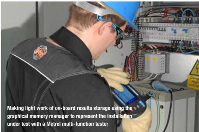
Making light work of on-board results storage using the graphical memory manager to represent the installation under test with a Metrel multi-function tester
